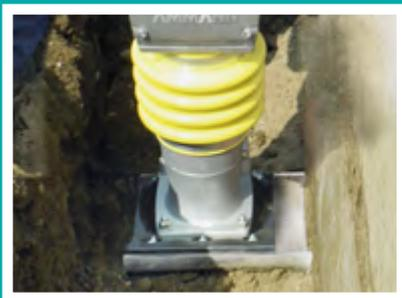
340 mm asymmetric: compaction work in trenches protected by shuttering systems: no need to inclining the rammer during operation.
